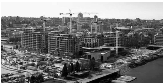
The Olympic Village Under Construction
